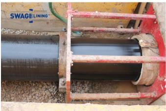
During the Swagelining<sup>™</sup> process the HDPE pipe is temporarily reduced as it is pulled through the reduction die.
